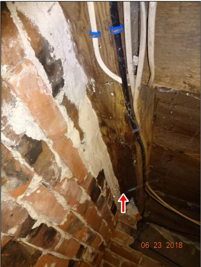
4.1 Item 3(Picture) old sill damage just inside crawl
