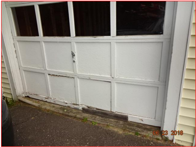
14.0.A Item 1(Picture) damaged door (1 of 2)
