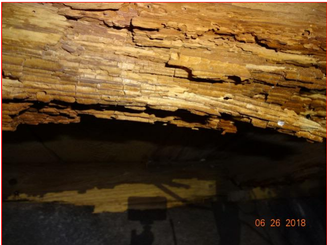
15.0 Item 6(Picture) Decayed joist
