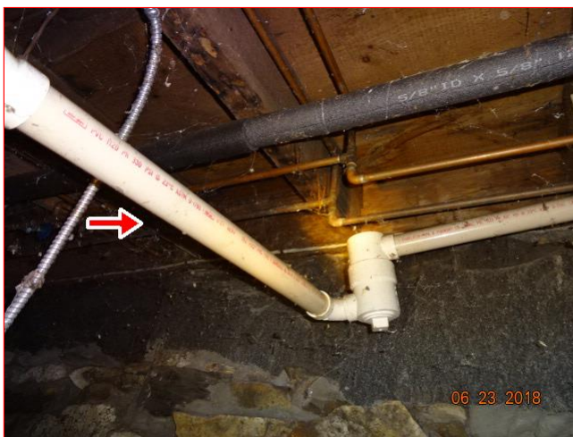
10.3 Item 1(Picture) direction of water flow front laundry drain
