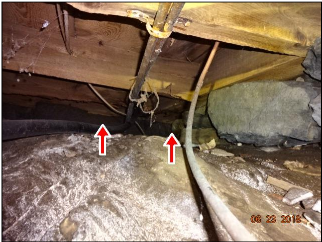
4.1 Item 2(Picture) area of suspected sill and beam damage.
