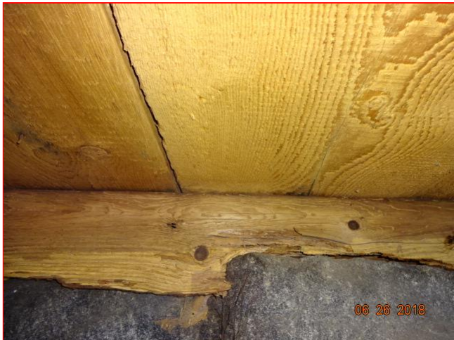
15.0 Item 3(Picture) Crushed sill at back wall
