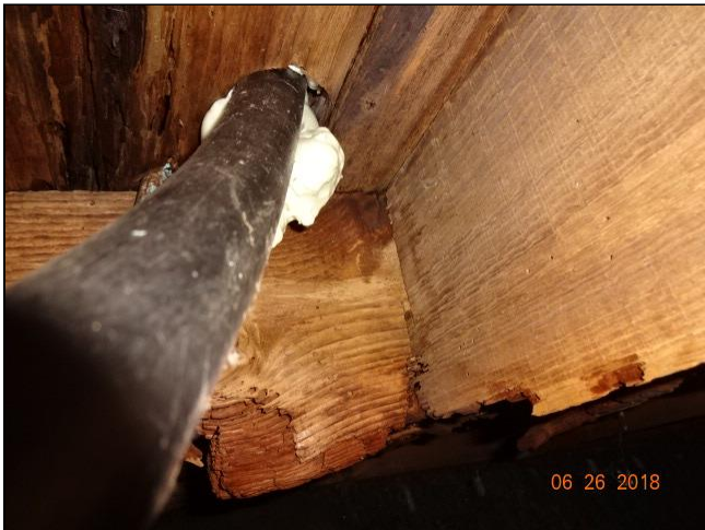
15.0 Item 5(Picture) Damaged joists and subfloor at washer drain
