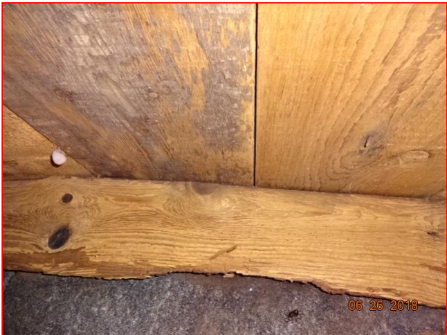
15.0 Item 4(Picture) Crushed sill at back wall
