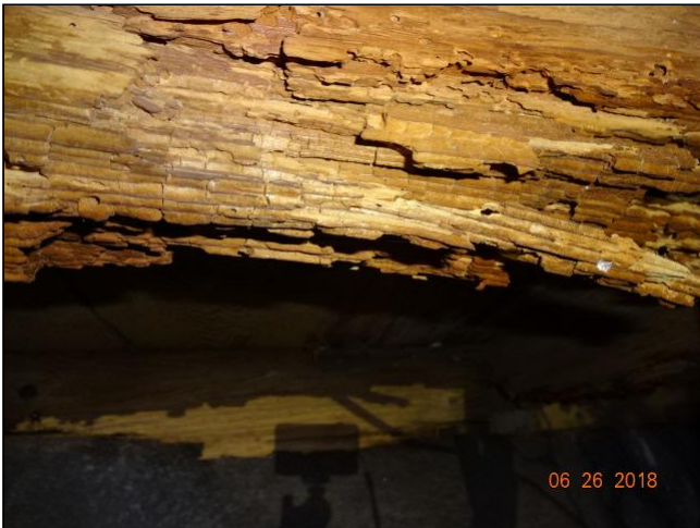
15.0 Item 6(Picture) Decayed joist
