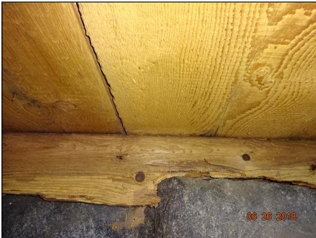
15.0 Item 3(Picture) Crushed sill at back wall
