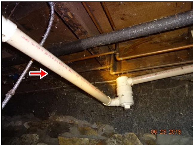
10.3 Item 1(Picture) direction of water flow front laundry drain
