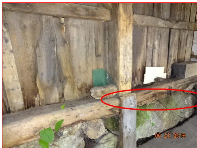
14.2.B Item 1(Picture) damaged sill
