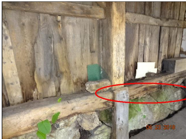
14.2.B Item 1(Picture) damaged sill
