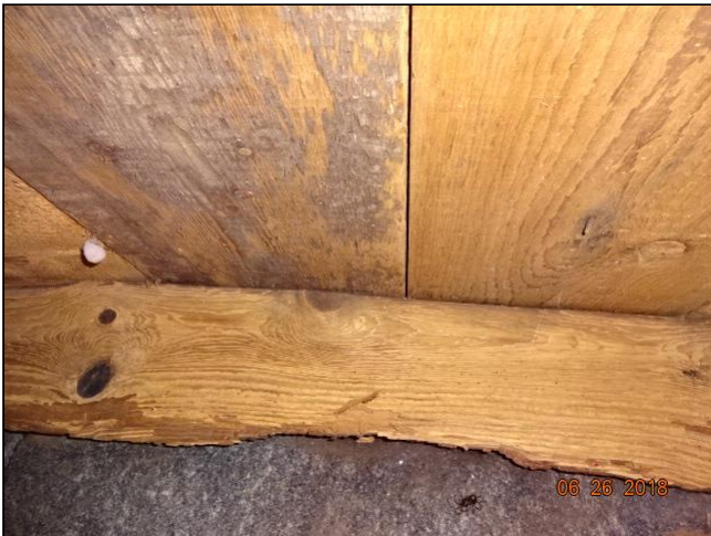
15.0 Item 4(Picture) Crushed sill at back wall
