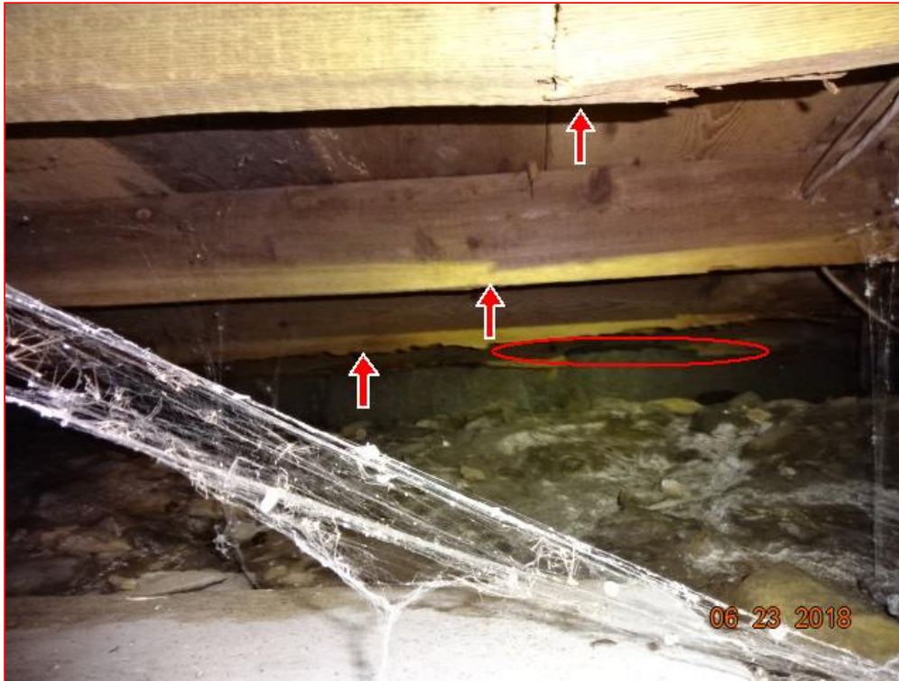
4.1 Item 1(Picture) damaged joists and possible bad sill (circled)
